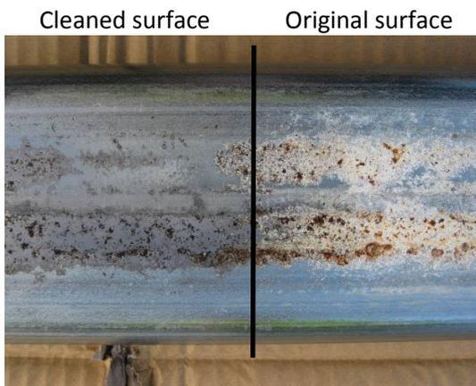
**Picture 2. White rust repair using Vinegar and nylon scourer**
