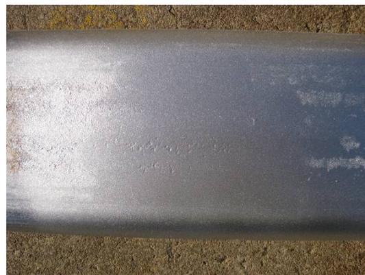
**Picture 5. Zinc paint repaired (wire brush wheel)**
